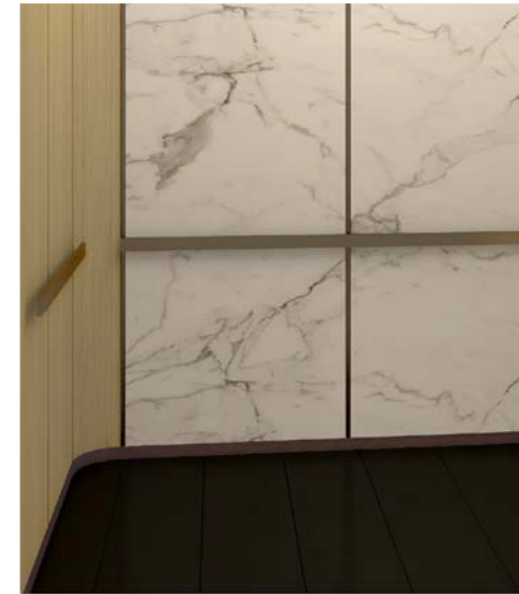
■ Ceiling: Drop Ceiling in PCF White, Hafele LED Striplight. ■ Wall: Back Wall in White Calacatta Stone with Natural White Oak Veneer
